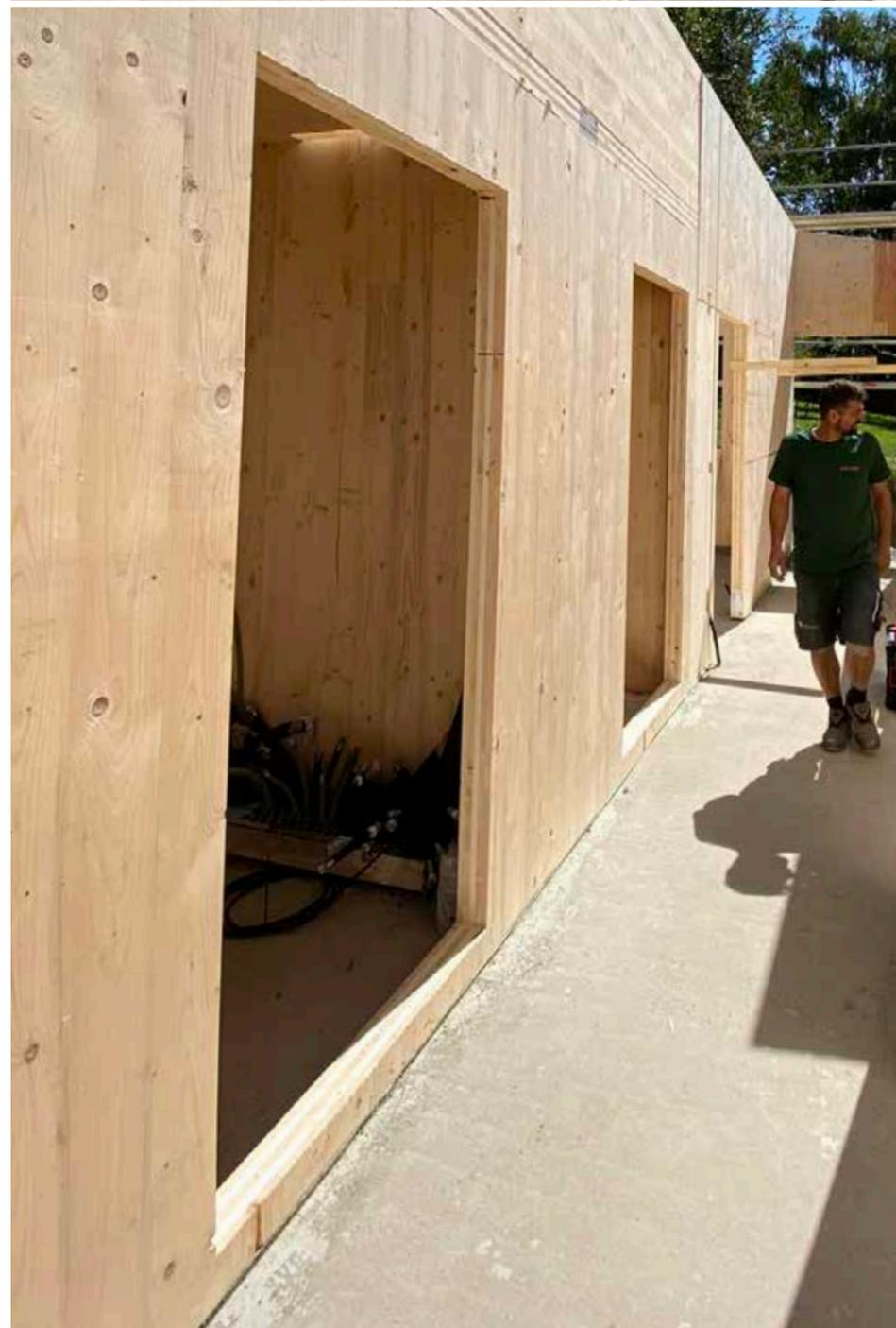
XWORKS buildings are fully pre-fabricated at the plant for dry assembly on site to ensure they do not transfer any additional moisture into the structure. The design does not include a diffusion barrier, so the walls can absorb the humidity in the room and evenly disperse it for a much nicer indoor climate.
